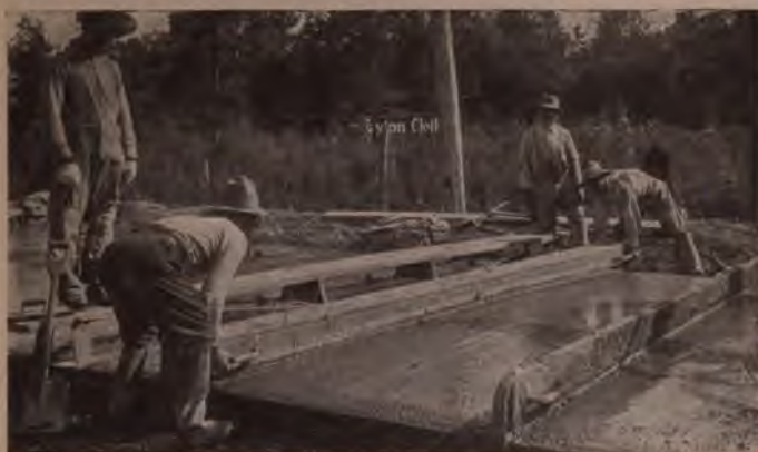
Striking Off the Surface.
